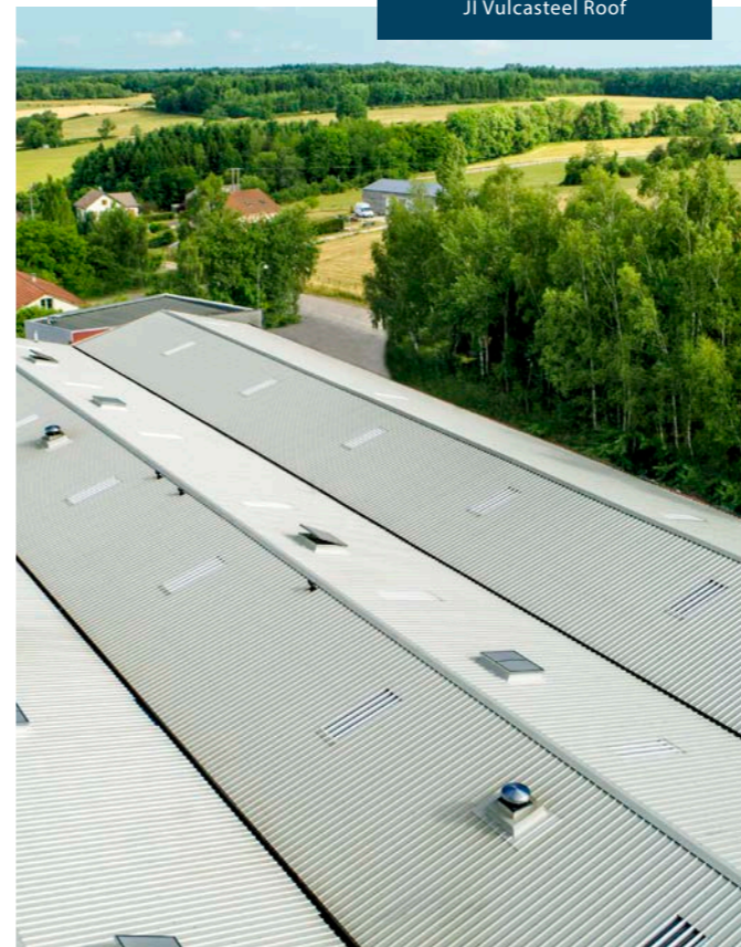
Jl Vulcasteel Roof
