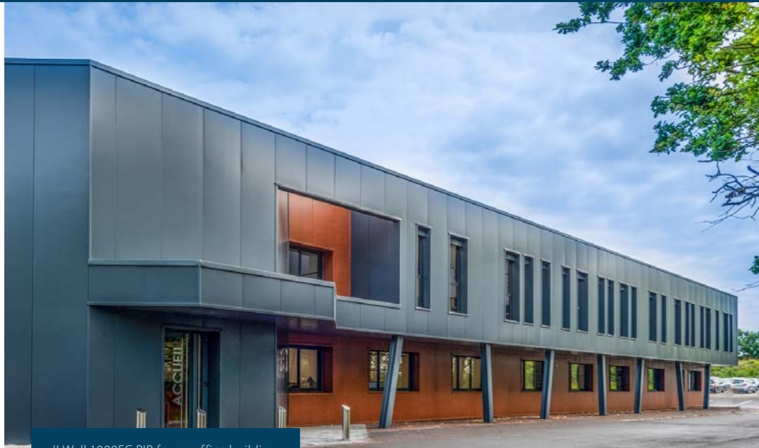
Jl Wall 1000FC PIR for an office building.
