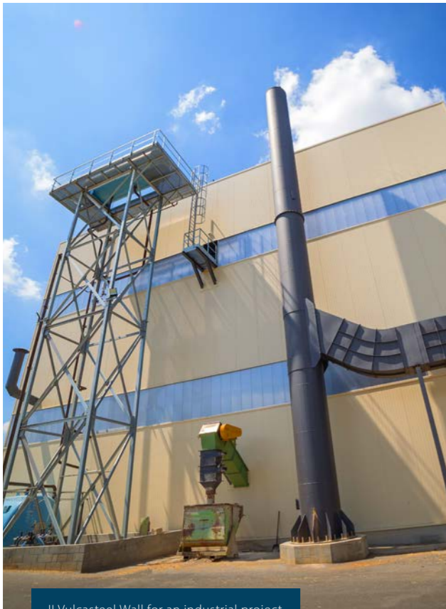
Jl Vulcasteel Wall for an industrial project.
